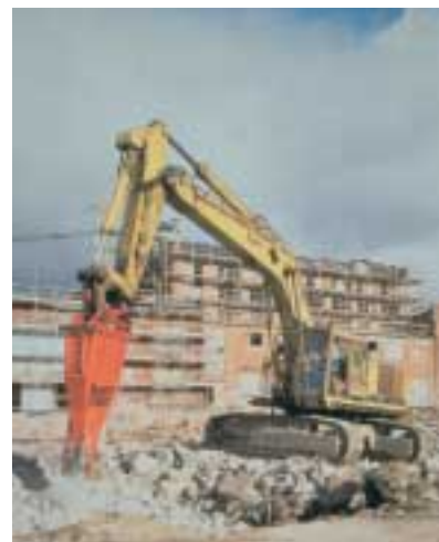
Rammer's hydraulic hammers are used in breaking and demolition, primarily in the construction industry.
